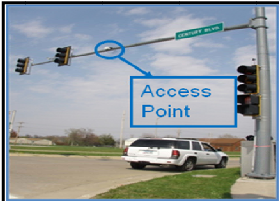
B - Detail access point.
