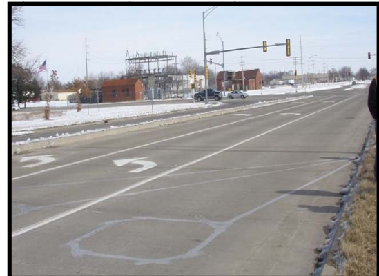
C - Eastbound approach.
